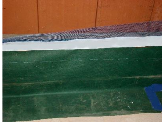
Figure 22. Non- adhesive membrane (glued on the vapour retarder) equipped with a grid to receive plaster against interior wall. Courtesy Wienerberger.
