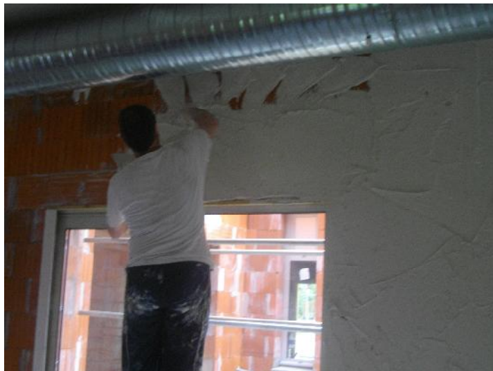
Figure 21. Plaster applied on interior wall.
