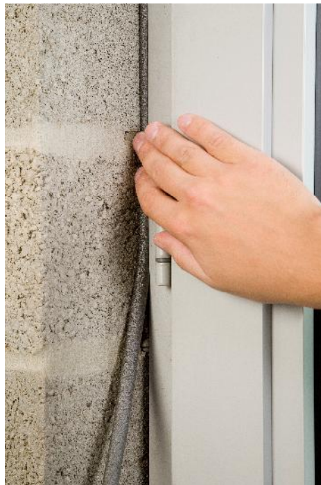
Figure 29. Closed-cell PE round backer rod. Courtesy Soudal.
