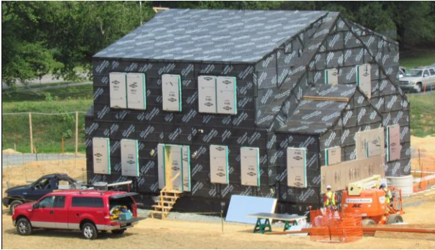
Figures 8 & 9. Construction of NZERTF showing the air barrier (left) and completed structure (right) (Ng, Persily & Emmerich, 2015).
