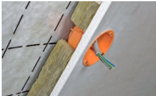
Figure 10. Space left behind gypsum board to allow electrical cabling to pass without perforating the airtight layer. Courtesy Isover.
