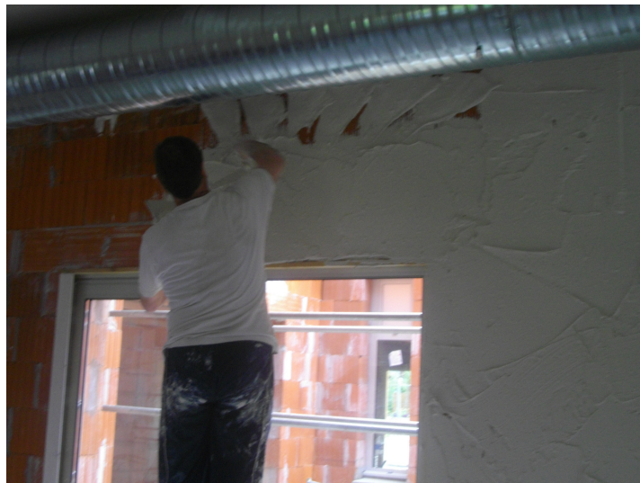
Figure 21. Plaster applied on interior wall.
