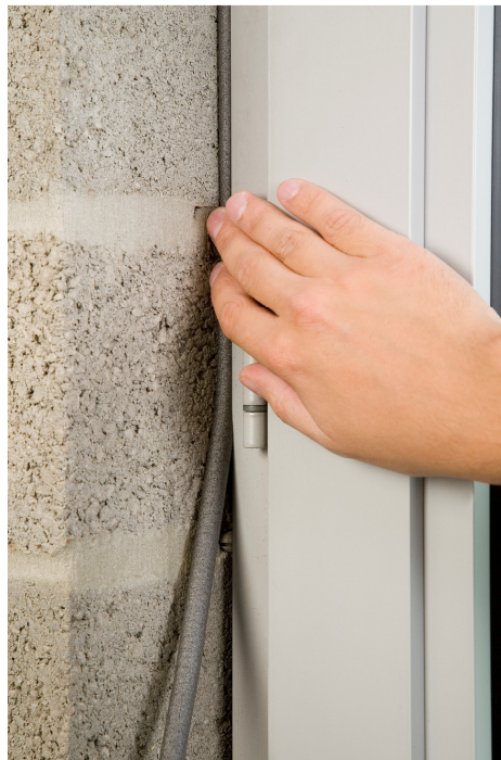
Figure 29. Closed-cell PE round backer rod. Courtesy Soudal.
