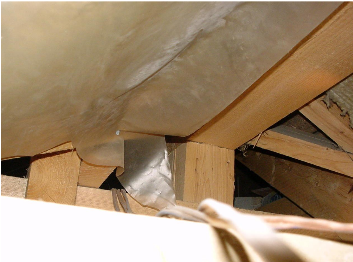
Figure 1: Building airtight means taking care of the connections!
